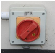
Typical Isolator Switch
